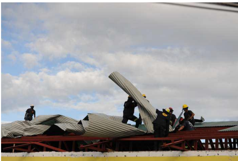
Figure 15: ESD personnel removing a roof of a hospital
